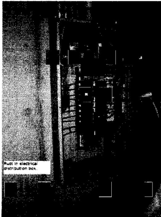
Any rust in the panel is a sign of water leakage. It is unsafe and a code violation.
