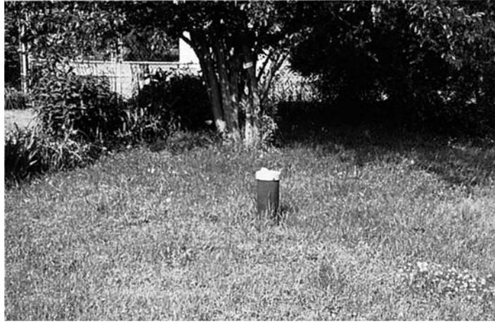
NOTE 1—Photograph shows an approximately 8-in. diameter outer well casing in the yard of a home. Releases of chemicals or petroleum products near or into a well can result in the contamination of the groundwater aquifer in which the well is constructed.
