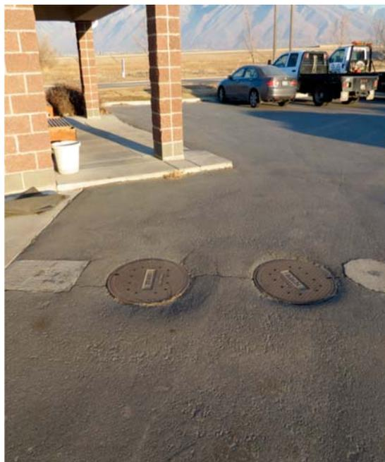
**FIG. X1.4** Manhole covers outside a vehicle repair shop leading to a two-stage oil-water separator. Oil-water separators are often located under manholes inside or outside repair garages, oil change facilities, restaurants or at any location where it is necessary to separate oil from water prior to discharge of the water to the sanitary sewer system, an on-site septic system, or to surface waters.
