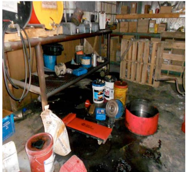
FIG. X1.10 Staining on the concrete floor from improper storage and dispensing of petroleum products. Heavy staining like this may indicate repeated leaks or spills that could migrate through the concrete to the underlying soils.
