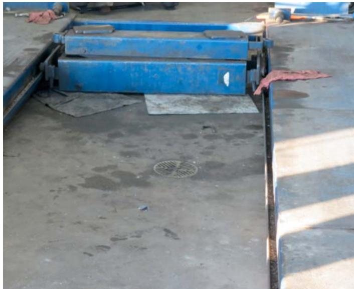
NOTE 1—Floor drains come in various shapes and sizes. Floor drains may lead to the sanitary sewer, the storm sewer, an oil-water separator, an on-site drain field/septic system, surface waters, or discharge directly into the ground below the drain. It is important to know the point of discharge of any floor drain in order to determine if the liquids reaching the floor drain are being properly disposed.
