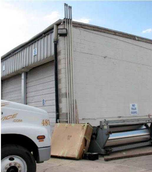
FIG. X1.8 Four vent pipes attached to the exterior wall of a commercial building indicating the presence or former presence of four underground storage tanks nearby.
