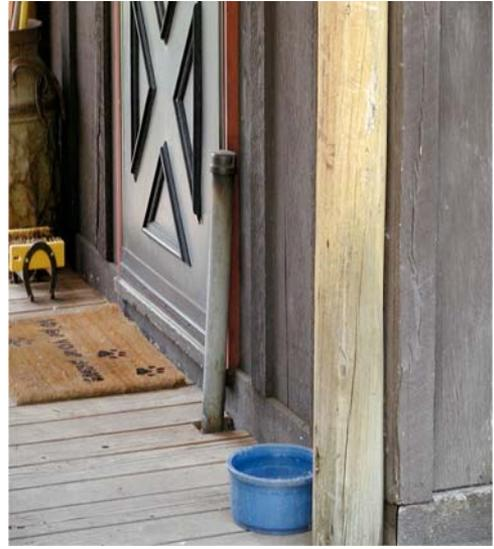
FIG. X1.9 Fill pipe for an underground storage tank containing fuel oil located on the back porch of a single family home.
