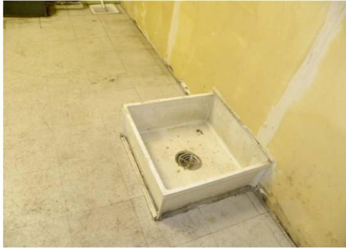
NOTE 1—Floor drains come in various shapes and sizes. Floor drains may lead to the sanitary sewer, the storm sewer, an oil-water separator, an on-site drain field/septic system, surface waters, or discharge directly into the ground below the drain. It is important to know the point of discharge of any floor drain in order to determine if the liquids reaching the floor drain are being properly disposed.
